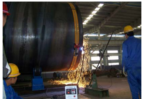
Plasma cutting, V-type bevel Pipe size dia 3740mm, wall thickness 22mm, spiral seam pipe
